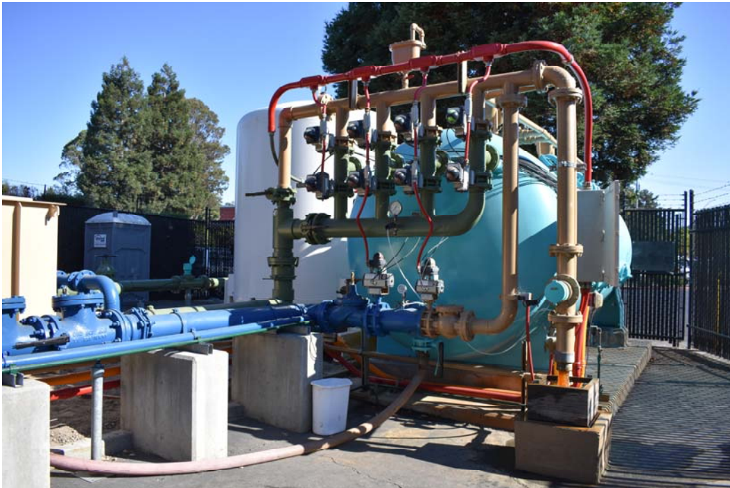
Your money at work – Well 10A after rehabilitations
