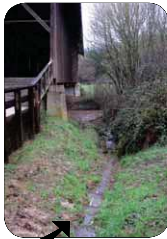
...AND CONTINUES DIRECTLY TO THE SAN LORENZO RIVER.
