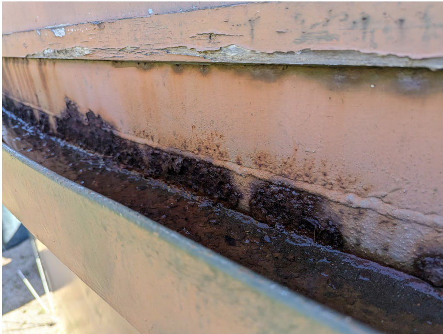
Photo 19 – Corrosion in the Roof Top Girder/Gutter
