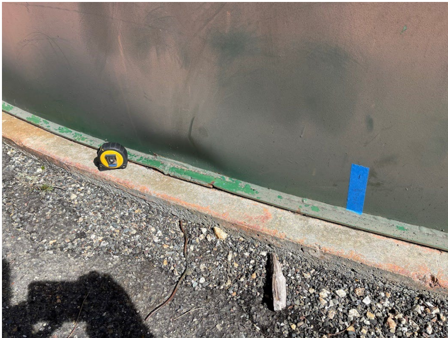
Photo 25 – "Dent" at Shell to Bottom Joint
