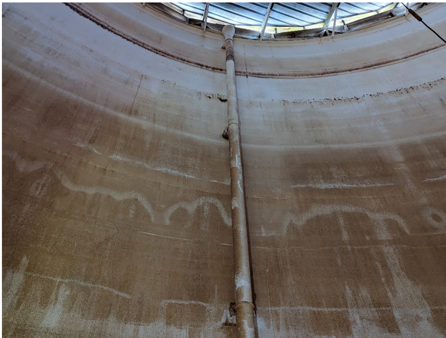
Photo 13 – Overflow up the shell
