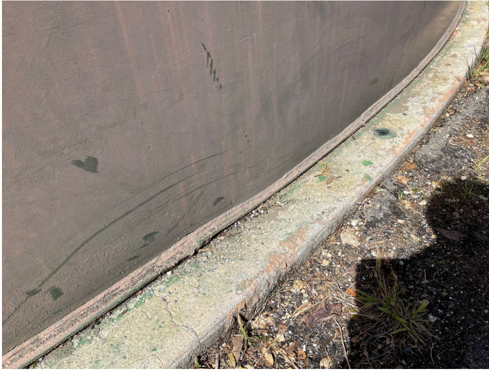
Photo 20 – Bottom Plate Projection. In this photo, the bottom plate projection varies greatly from the bottom left to the top right. There appears to be three welding passes in some areas, where only one should have been used.
