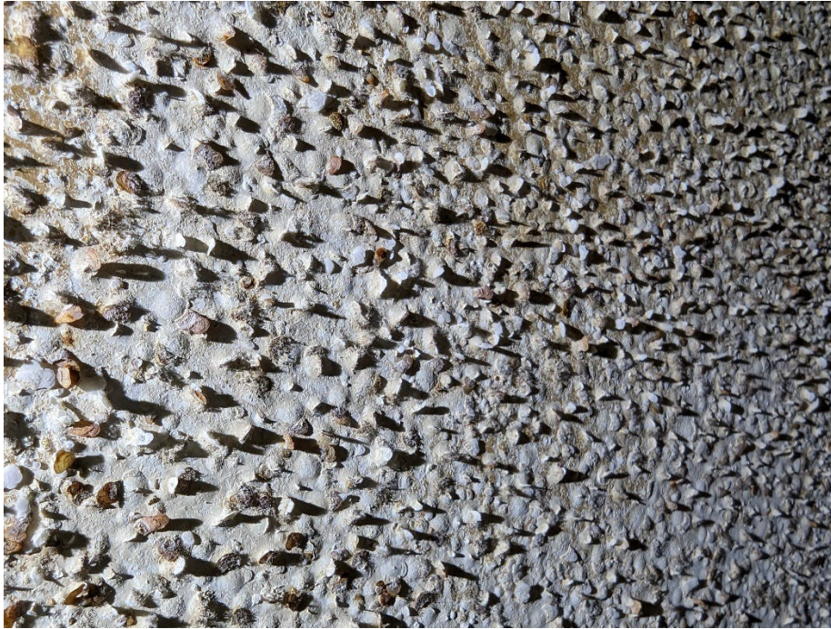
Photo 4 – Closeup of Shell Coating Blisters
