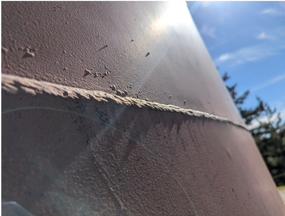
Photo 21 – Weld Splatter on Horizontal Joint, Ring 1 to Ring 2
