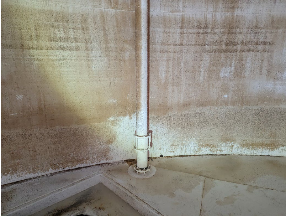
Photo 12 – Overflow at Bottom
