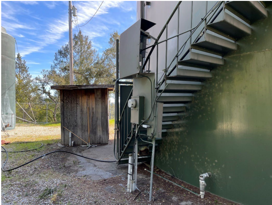
Photo 24 – Rear View of Stairway. Note the lack of overlap between treads and presence of a toe board at rear of each tread.
