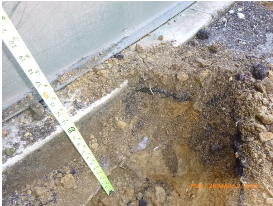
Photo 30 – Foundation Appears to Be About 12 inches In Depth
