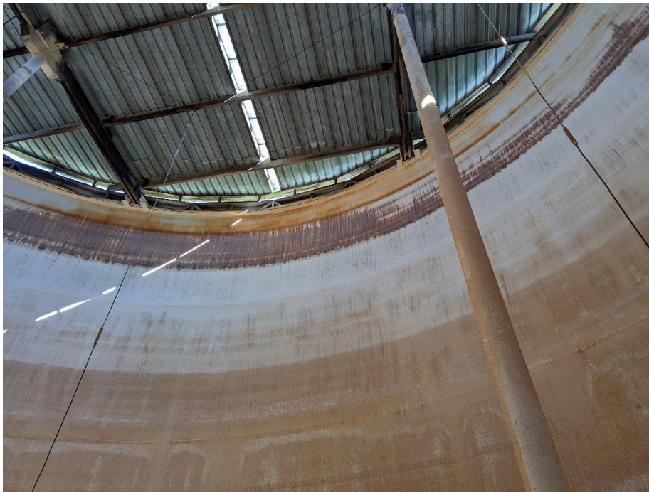
Photo 7 – Coating Failure and Corrosion Above the Operating Water Level
