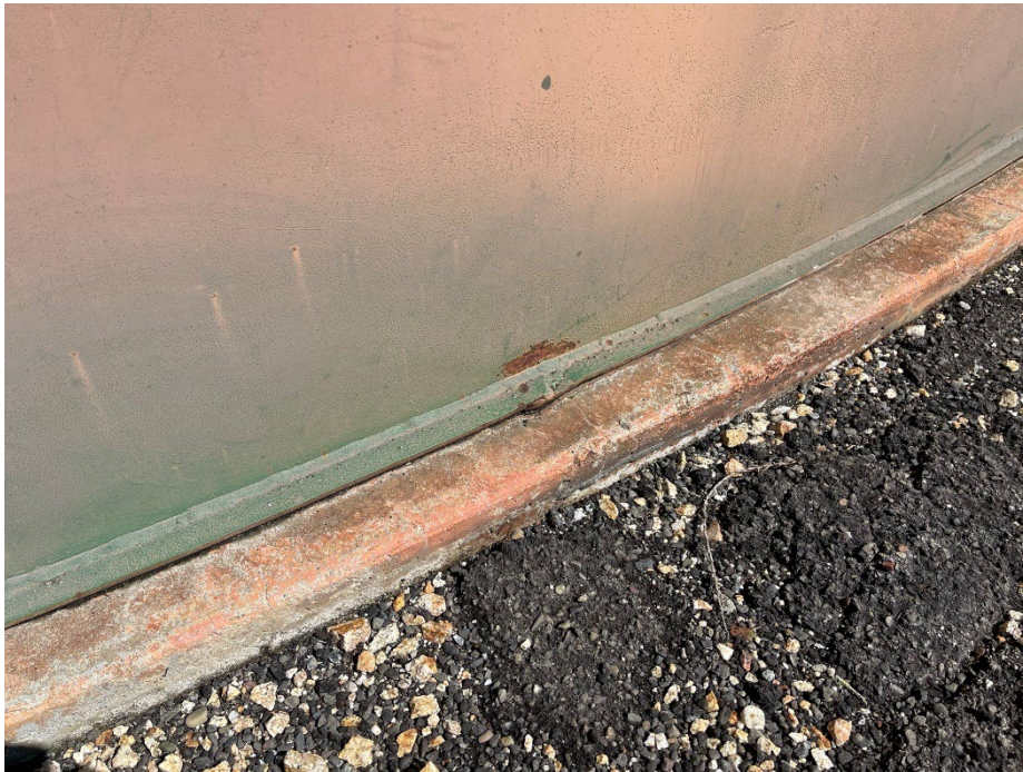
Photo 22 – Weld Repair at Shell to Bottom Joint
