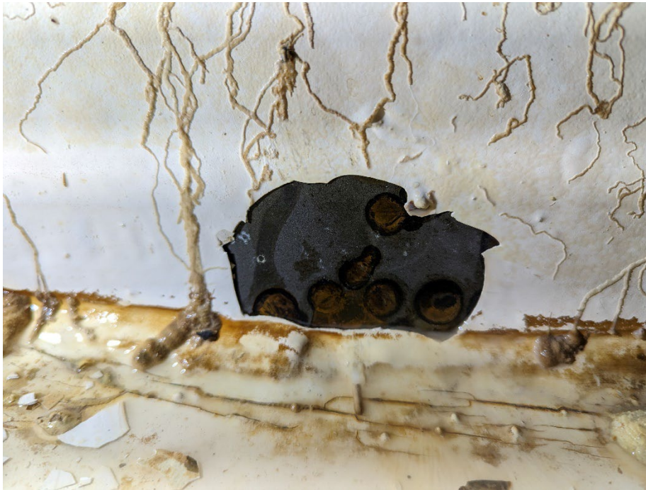
Photo 8 – Corrosion at Spalled Coating at Base of Shell. Cathodic protection system is limiting the depth of corrosion pits.
