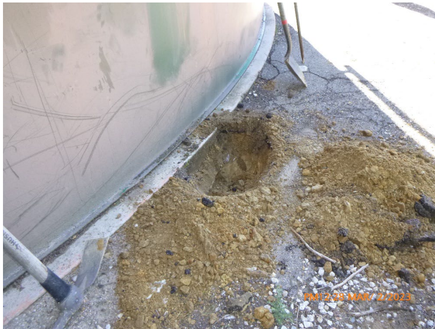
Photo 29 – Excavation for Depth of Concrete Foundation
