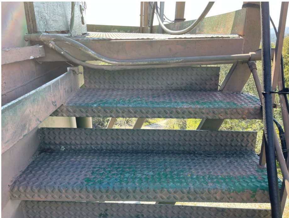
Photo 23 – Stairway Tread. Note the toe board at the back of the treads.
