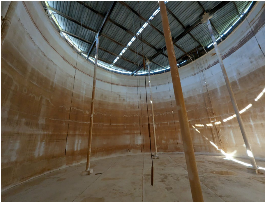
Photo 1B – Interior View. Showing the columns, roof, and cathodic protection anodes
