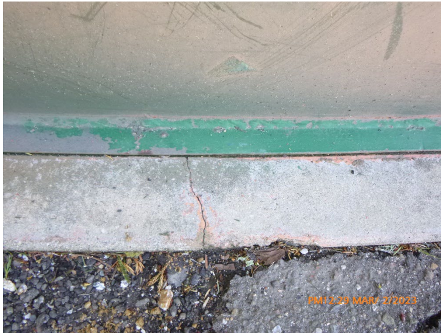
Photo 27 – Radial Crack in Concrete Foundation
