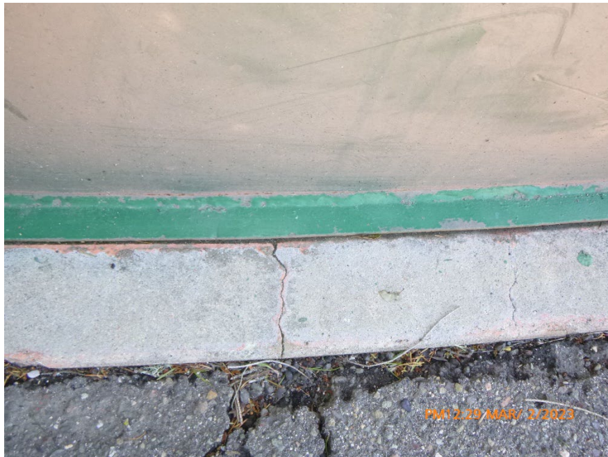
Photo 28 – Radial Cracks in Concrete Foundation. There are two cracks in this photo.
