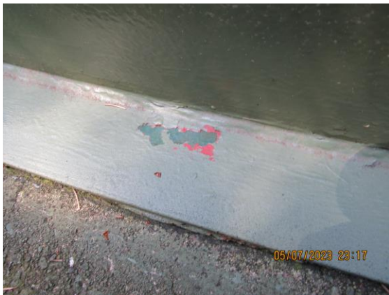
Detachment of over coat at floor plate extension
