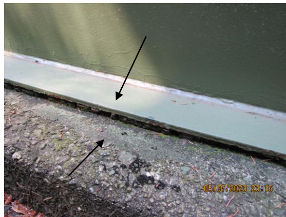
No caulking at interface between foundation and tank floor plate extension
