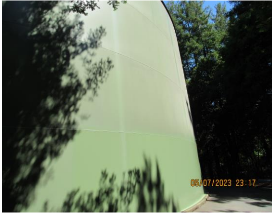
The exterior shell plate coating is in good condition.
