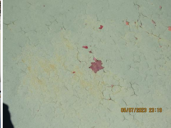
Failed fractured roof plate coating.
