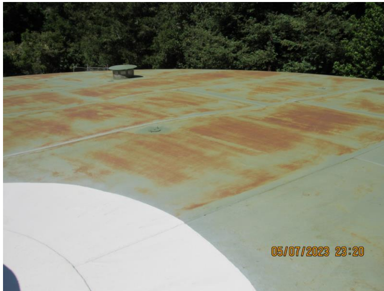
Failed fractured roof plate coating.
