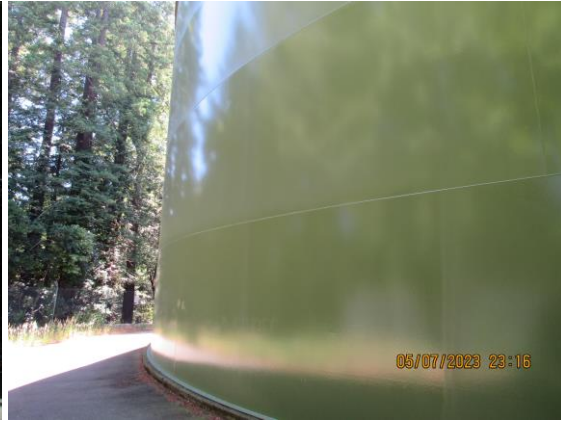
The exterior shell plate coating is in good condition.
